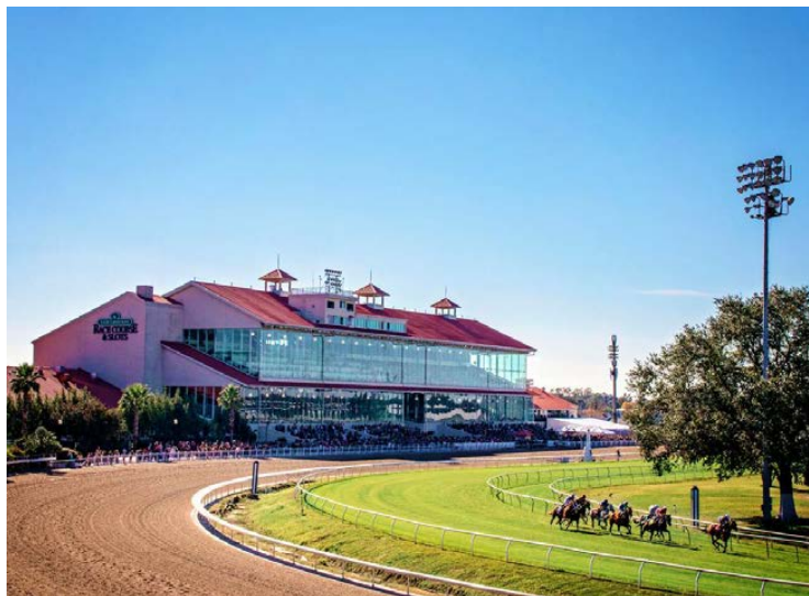
Racing at Fair Grounds in Louisiana | Hodges Photography
